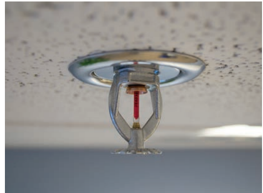
Figure 36. Fire sprinkler roof (ceiling) mount side view
