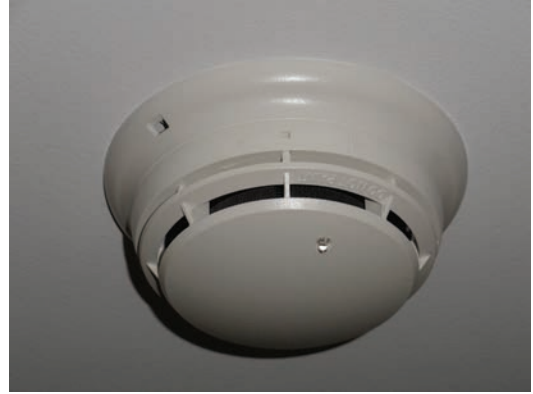
Figure 24. Smoke detector
