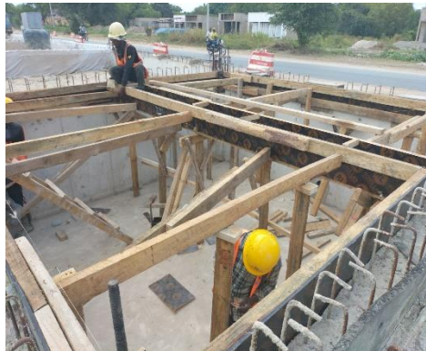
Photo 2: Construction of Gombo La Mboti Terminal
