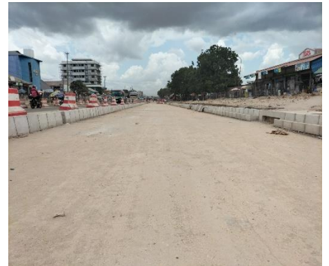
Photo 3: G15 layer on Mixed Traffic Lane
