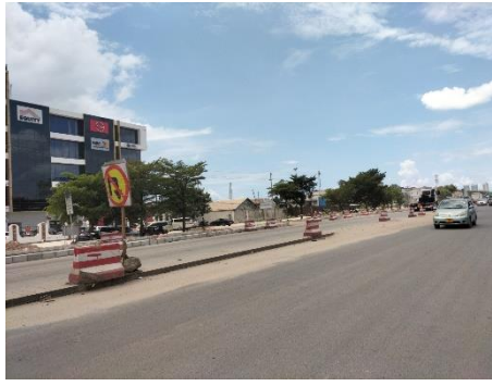
Photo 5: DBM layer Mixed Traffic Lane
