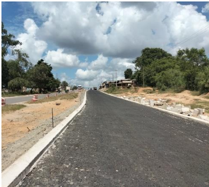
Photo 1: CRR laid on Mixed Traffic Lane
