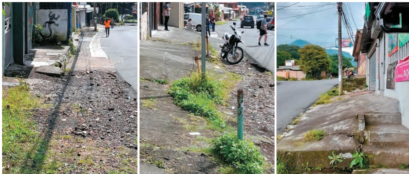
FIGURE 20. Street sidewalks in Aserri pose physical barriers
