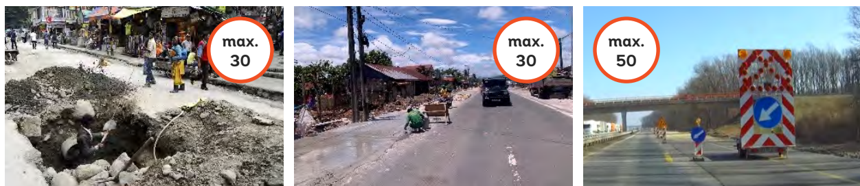
Figure 13. Typical examples of roadwork zones
