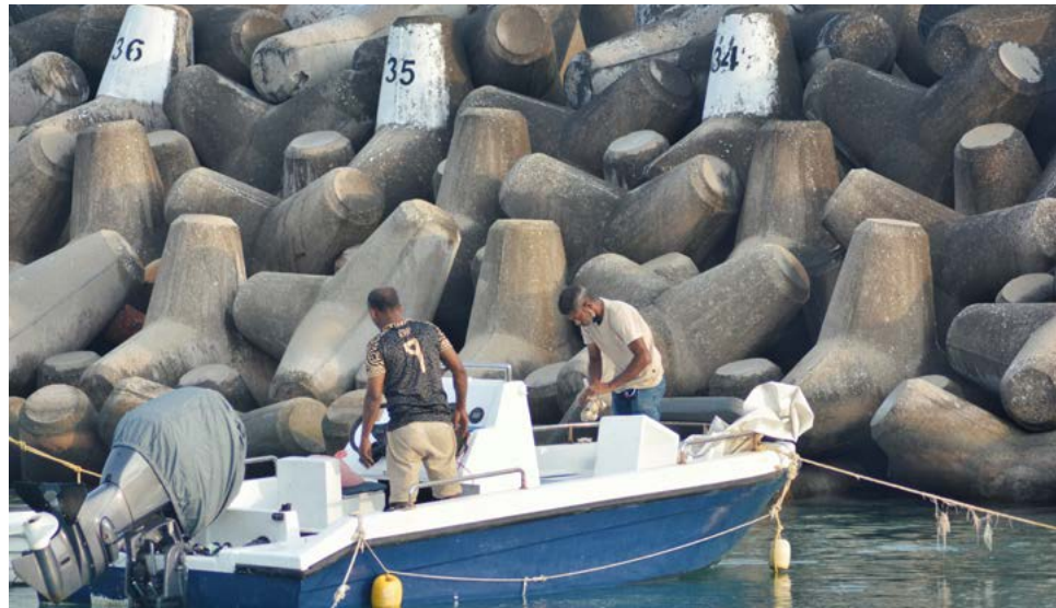
Photo Description: Concrete coastal protection around the Male City © World Bank
