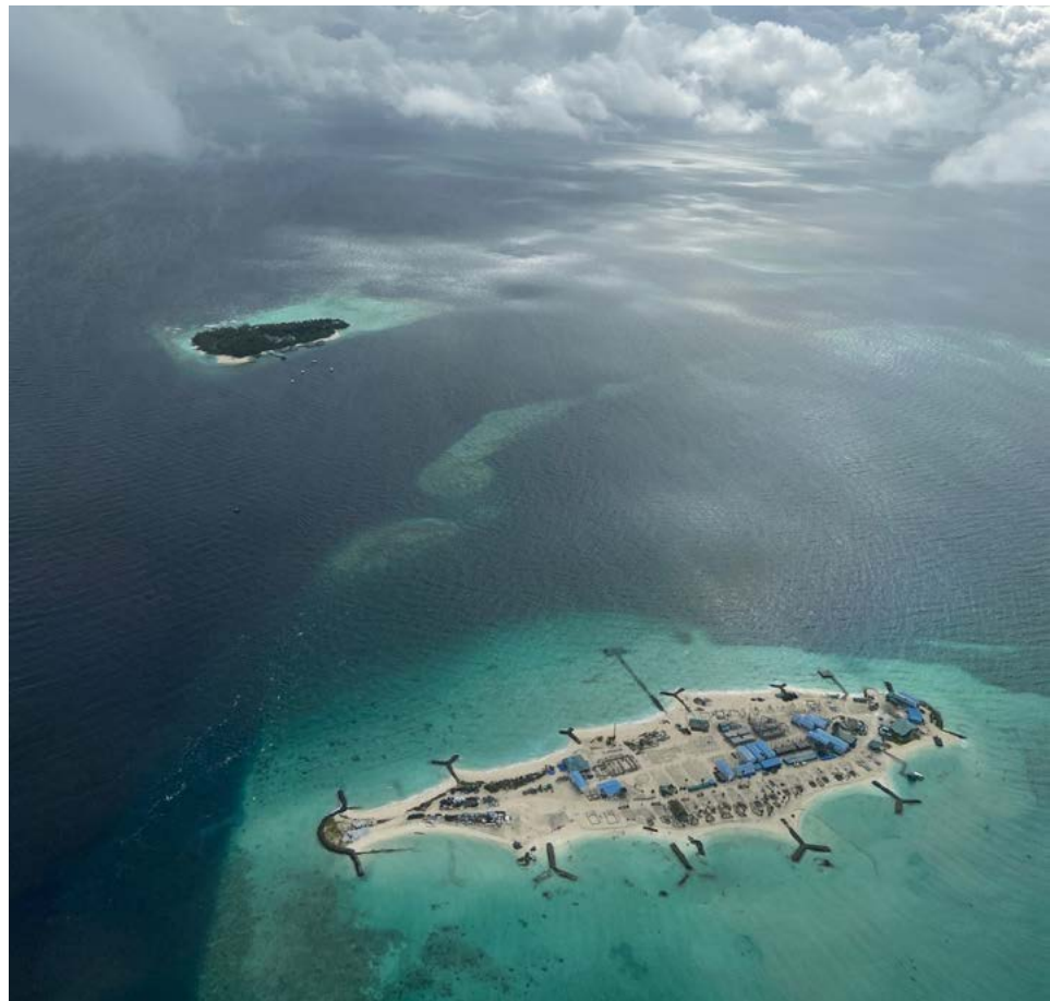
Photo Description: Aerial View of a Island Cleared and being Developed, Maldives © World Bank
