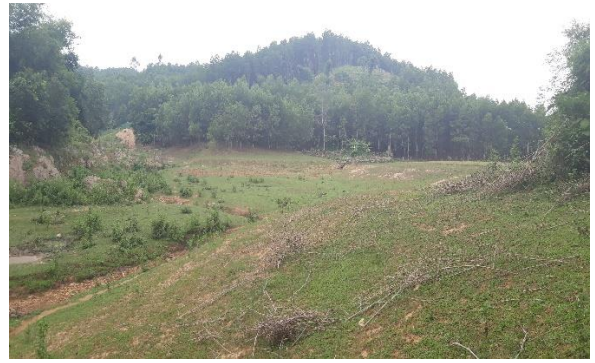
Spillway of Luong Bai Reservoir
