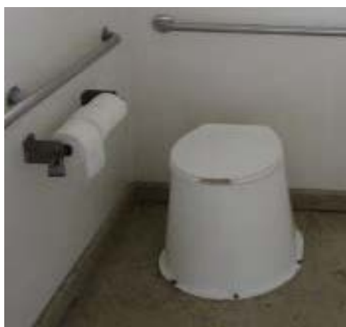
Photo 3.8 Pit Latrine with Improved User Interface
