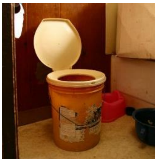
Photo 3.10 Typical In-House Bucket Toilet
