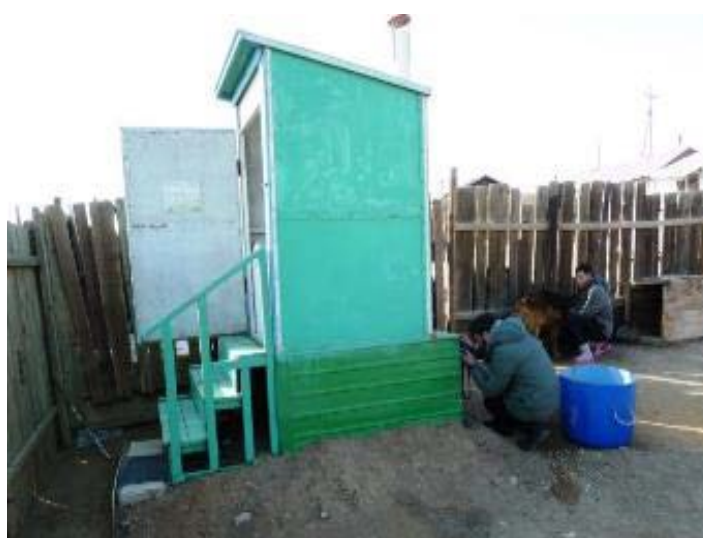
Photo A.5 Container-Based System with Urine-Diverting Dry Toilet in Ulaanbaatar, Mongolia
