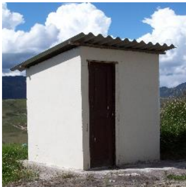
Photo 3.2 Latrine Superstructure, Ecuador
