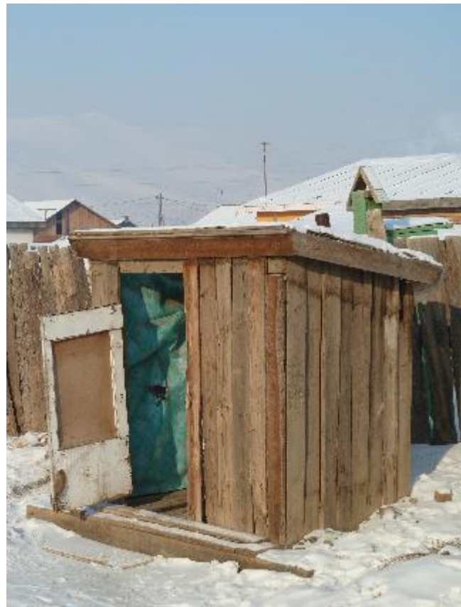
Photo 3.1 Typical Pit Latrine in Ulaanbaatar, Mongolia Source: World Bank.
