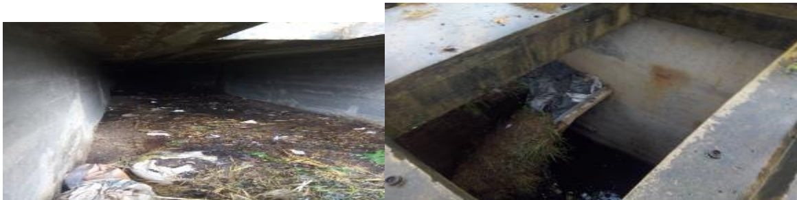
Figure 3.5: Abandoned site at Okpara mine CPS Ogbete Enugu
