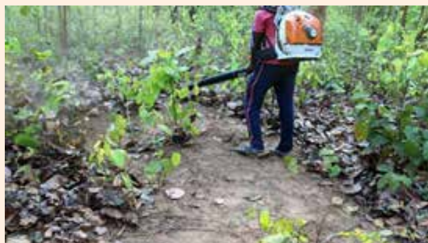
Fire line cleared of flammable litter
