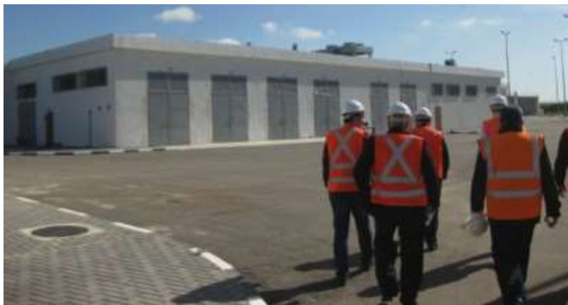
Figure 12-21: Outside of the blower and electrical building
