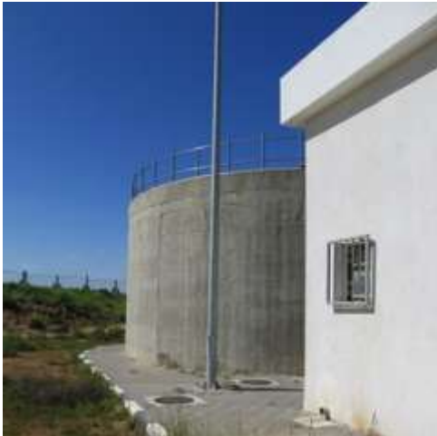
Figure 12-3: Backward of the Sludge Dewatering Building
