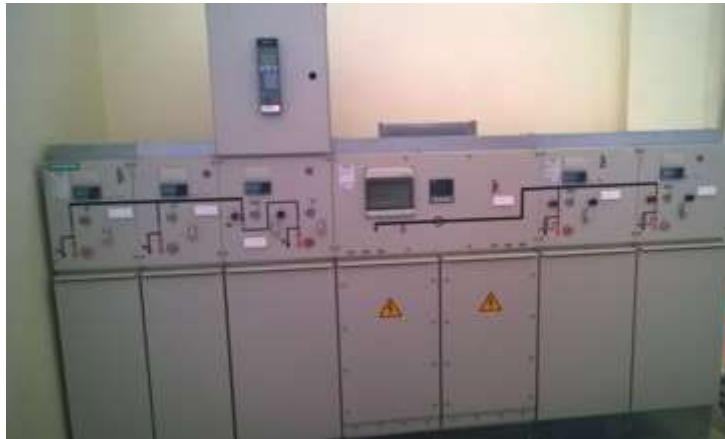
Figure 12-26: Ring-Main-Feeder switchgear
