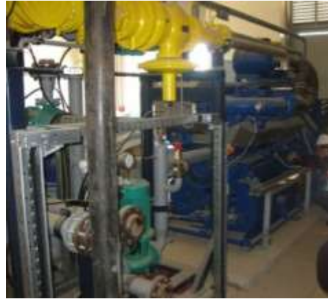
Figure 12-23: Biogas-engine
