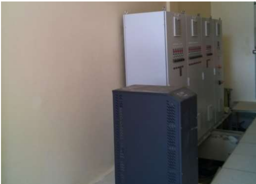
Figure 12-30: Cable trays and channels beneath the floor of the electrical room
