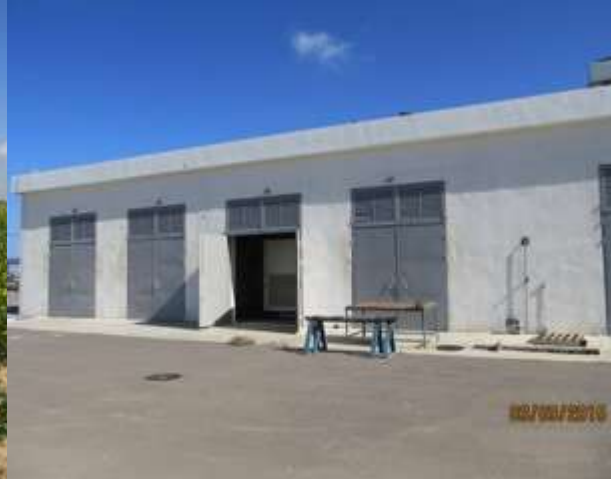
Figure 12-20: The Blower and energy building
