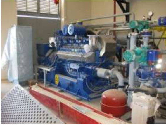
Figure 12-22: Biogas-engine
