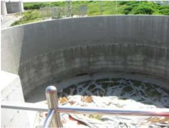
Figure 12-31: Future gas holder; storage Facility for biogas
