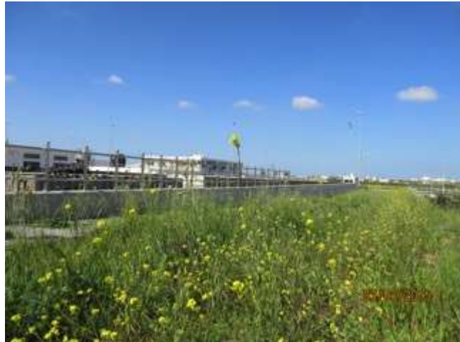
Figure 12-4: Embankment South of IB
