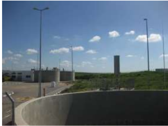
Figure 12-32: Flare near to the gas holder. Sludge silos in the background
