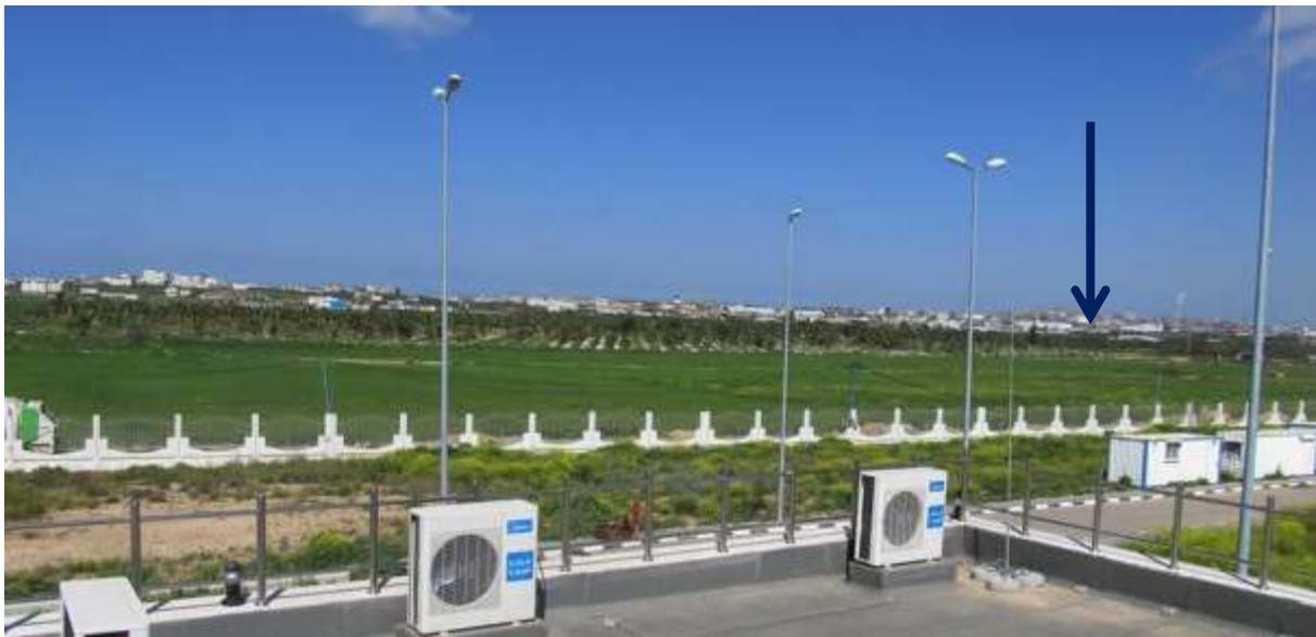
Figure 12-9: View from Administration Building towards the recovery scheme
