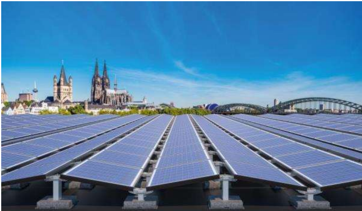
Figure 5-1: East-West orientation on a rooftop, press photo by manufacturer Renusol 33
