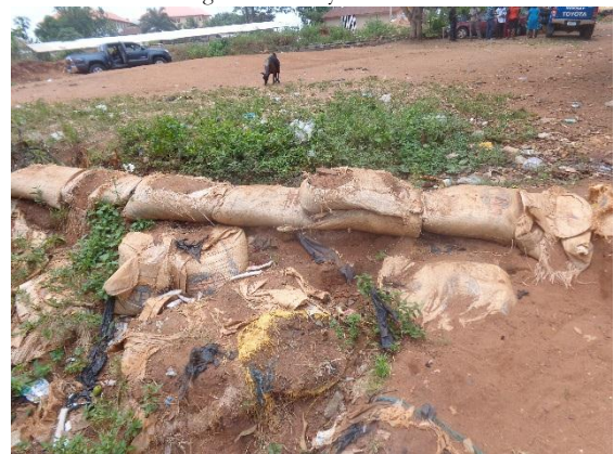
Figure 7 Embankments to control erosion
