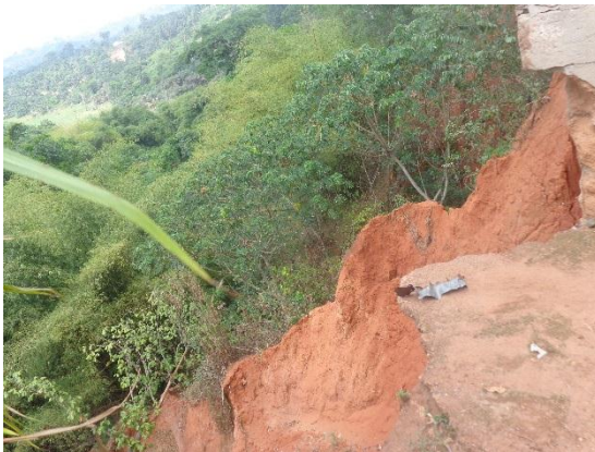
Figure 4 New land slide at the erosion site
