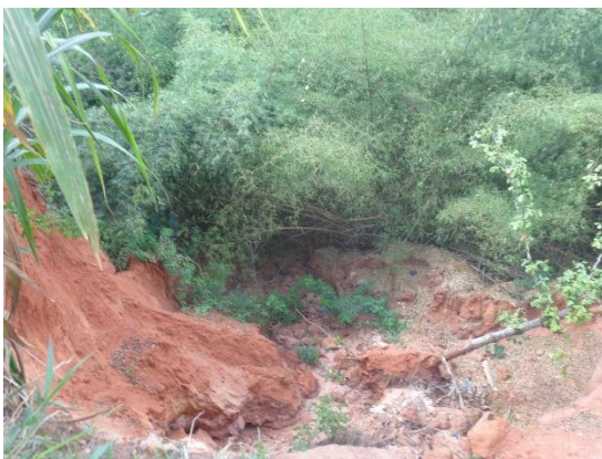
Figure 6 The Erosion site
