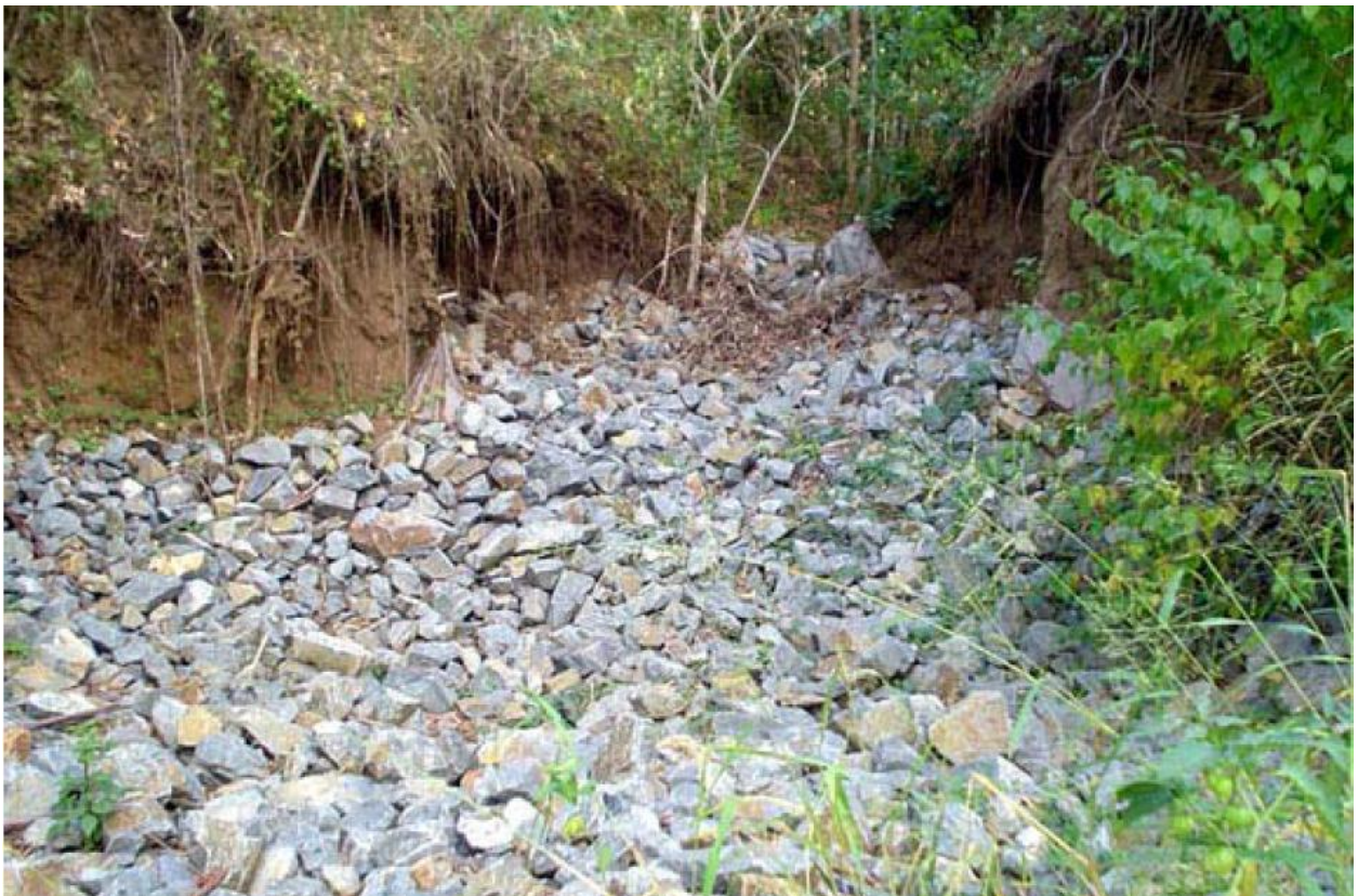
Figure 12 A Rock lined chute
