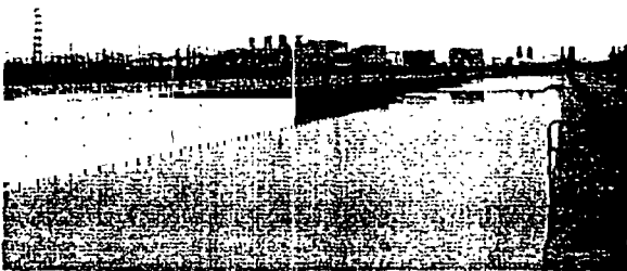
Intake canal looking towards the plant
