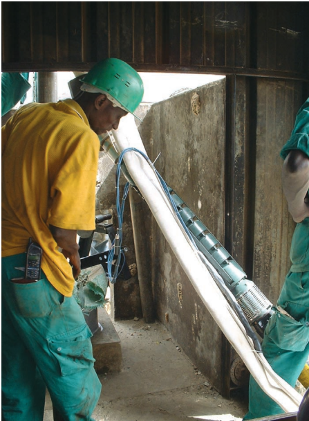
A private operator installing a water pump
