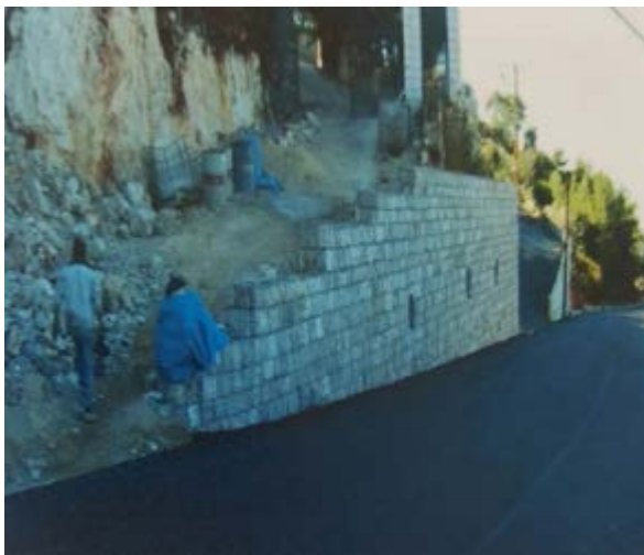
Saadiyyat Project - Masonry wall
