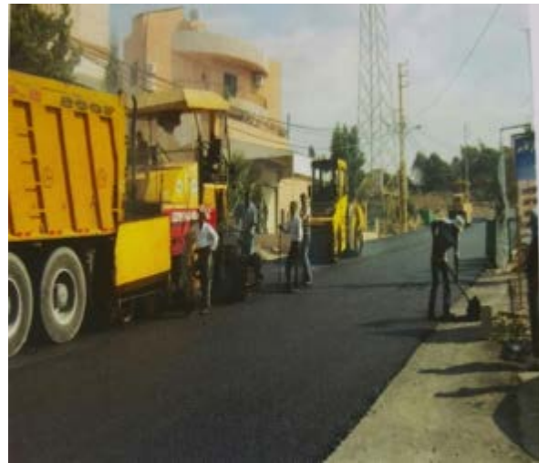
Saadiyyat Project - Asphalting works
