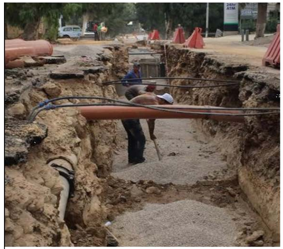
Hazmieh Project - Water and wastewater network
