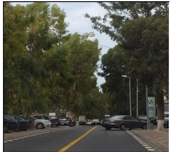
Hazmieh Project - Road after rehabilitation
