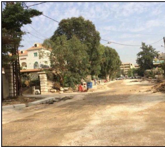
Hazmieh Project - Surface works
