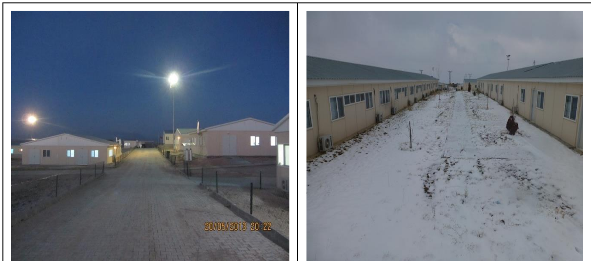
Picture 3.5.1. A view from campsite on Tuz Gölü Underground Natural Gas Storage Project (TG UNGSP) under construction.
