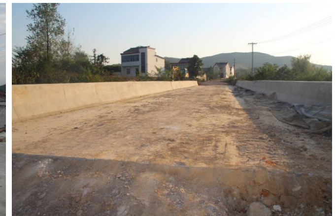
Dangerous Bridge Renovation, Shucheng 2015
