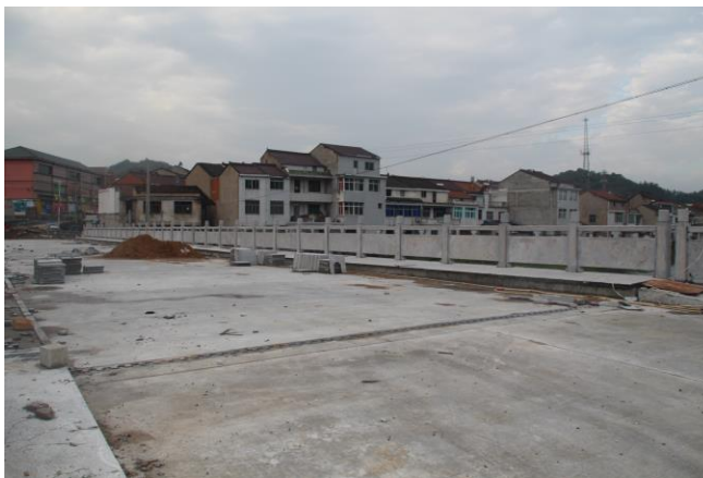
Dangerous Bridge Renovation, Shucheng, 2014
