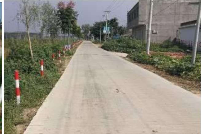
Road Safety Measures, Linquan, 2017
