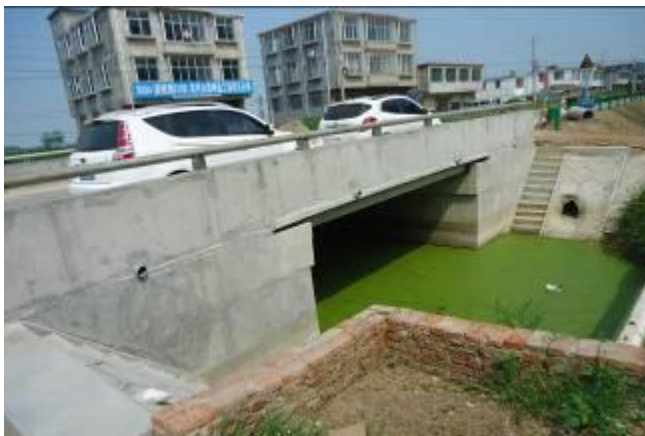
Dangerous Bridge Renovation, Xiaoxian, 2017
