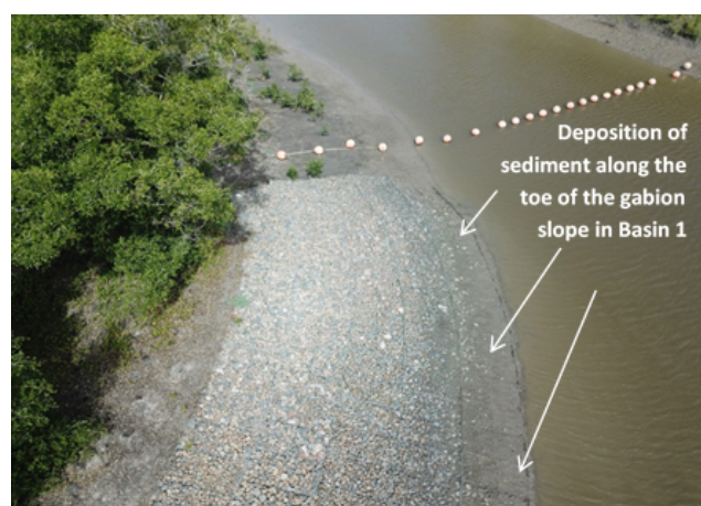
Figure 3-10 Deposition of sediment along the river July 2018
