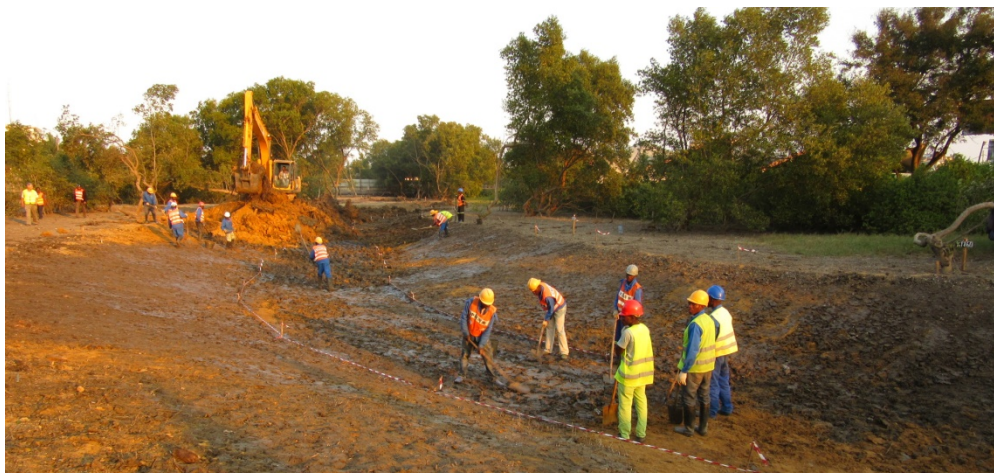
Figure 3-6 Excavation works in Basin 1. (Source: INROS LACKNER)
