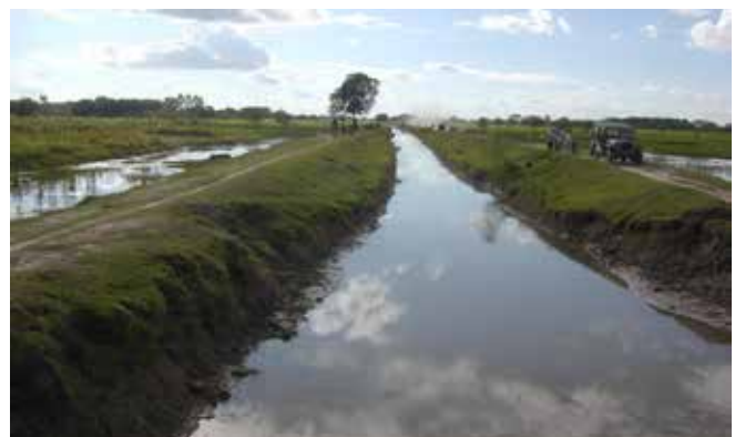
Figure 49 Waterlogging Along the Sarda-Sahayak Canal System in India
