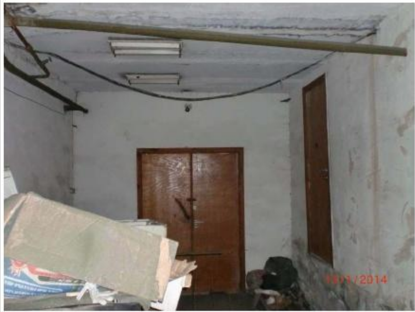
Main building basement, Side corridor (east side)
