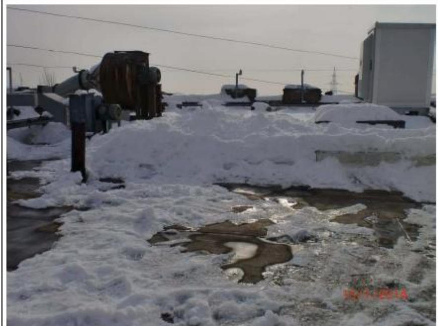
Main building roof, Flat roof with ventilation elements
