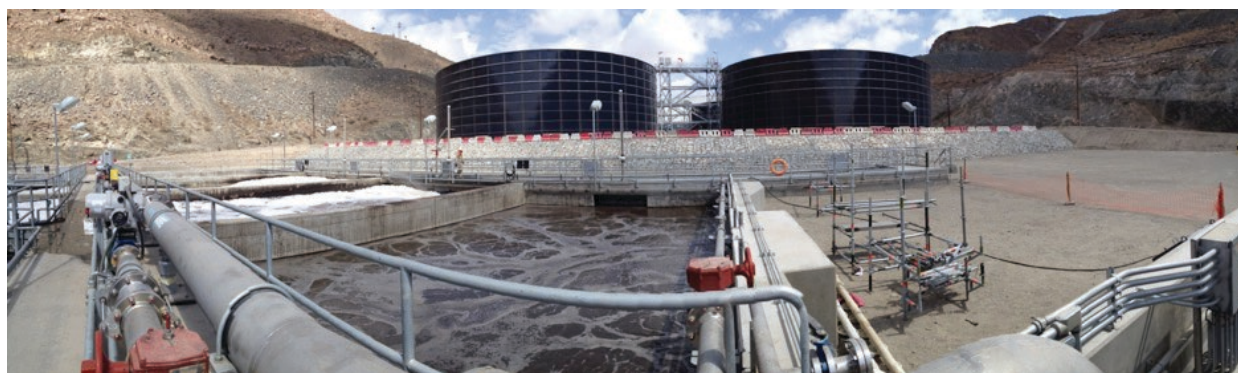
Panoramic view of the Enlozada wastewater treatment plant. Source: Photo by Daniel Nolasco, 2016.
