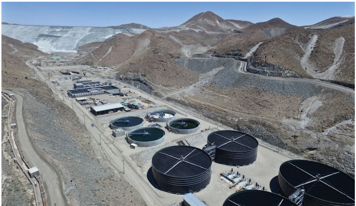
Aerial view of La Enzolada wastewater treatment plant. Source: Cerro Verde, 2018.
