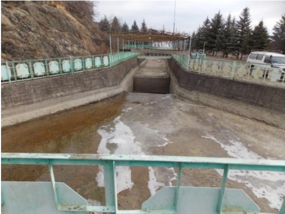
Discharge of the main canal
