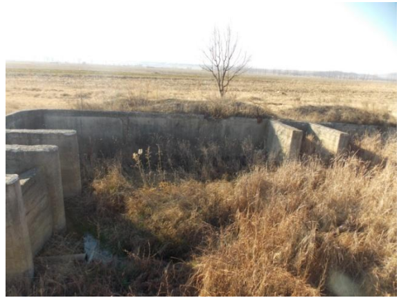
Reservoir adjacent to Koda-Marneuli motorway
