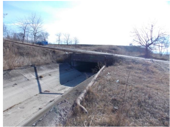
Shavsakdrisi canal crossing the motorway
