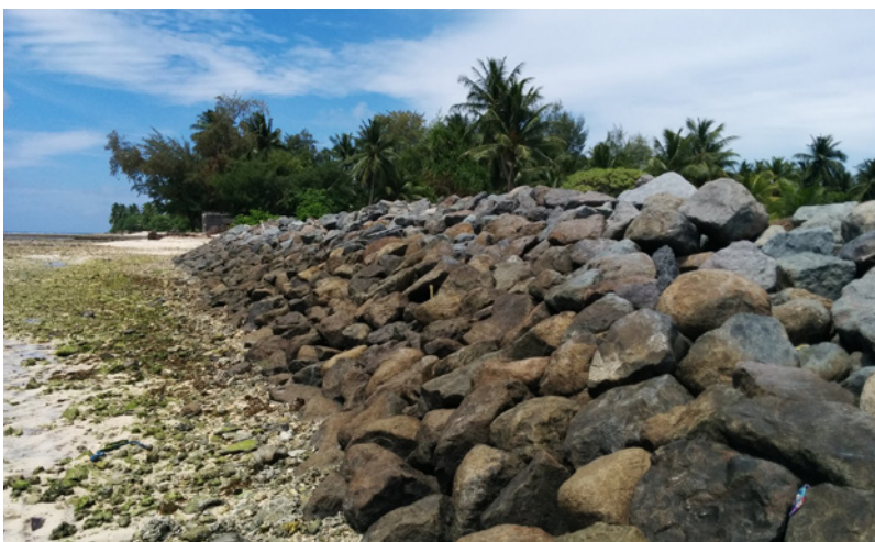
Figure C.10. Rock Revetment in Temaiku, South Tarawa
