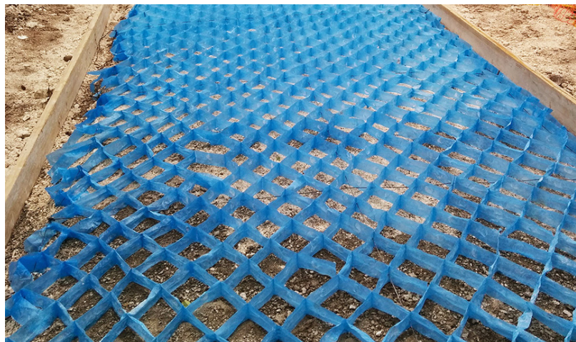
Figure C.8. Geocell Formwork Ready for Placement of Concrete
