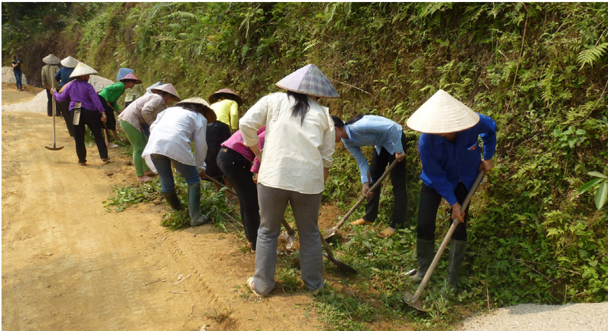
Figure 3.10. Construction of Road Drainage Systems by Local Communities in Vietnam
