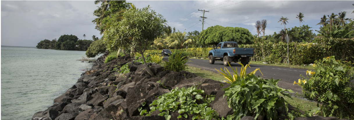
Figure 3.6. Samoa's Vulnerable West Coast Road
