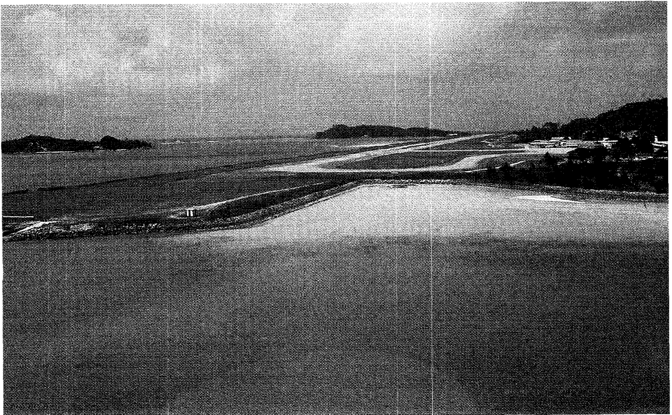
Land reclamation for airport in Mahé, Seychelles. (Photograph: Stefan Rosengren)
