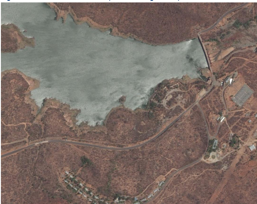
Figure 7. Mtera dam and reservoir (Source: Google Earth).
