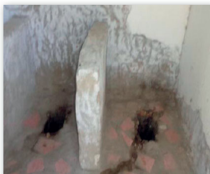
Photo 14. Toilet facilities at a college, Jizzak city
