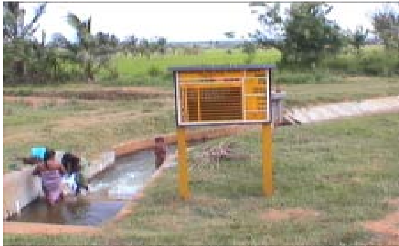
Figure 2: Display Boards fixed at calibrated outlet canal
