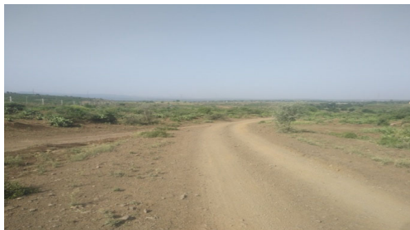
Figure 5.1.2-1: Gravel Road towards Mullu Town
