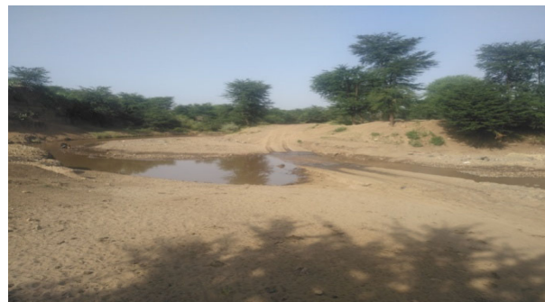
Figure 5.1.2-2: Meisso River Crossing, along the Gravel Road, KM 74+000
