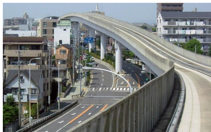
Figure 6-2. Elevated BRT Corridor in Nagoya, Japan
