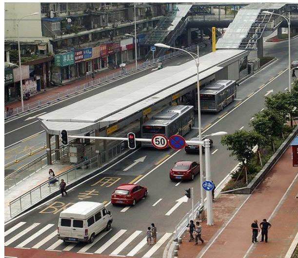
Figure 2-12. Median Bus Station
