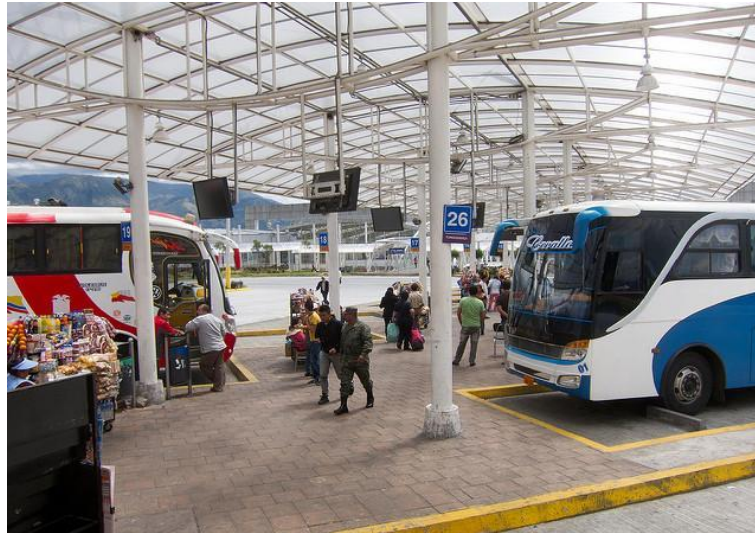
Figure 2-20. Bus Terminal in Quito, Ecuador
