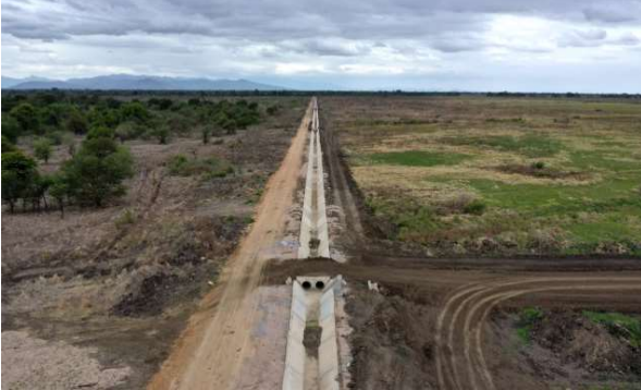
Main Canal 1 at Kilangali Seed Farm, Kilosa
