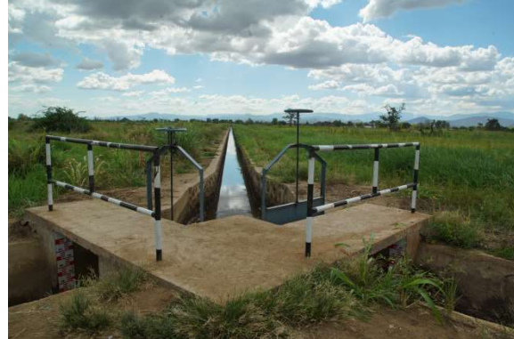
Division gates at Mvumi irrigation scheme, Kilosa
