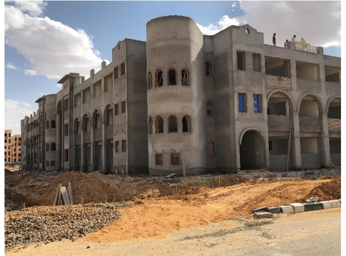
Figure 14: School under construction
