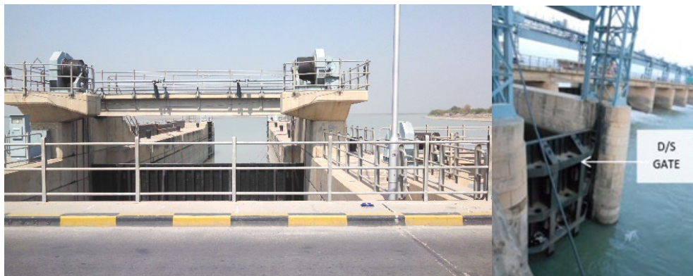
Figure 7: Ship-lock at Chashma Barrage
