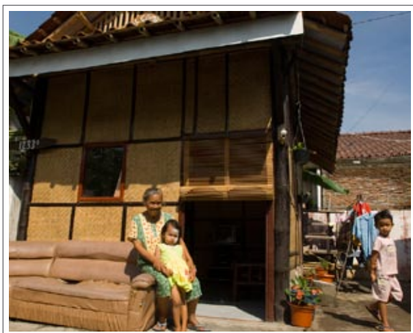
World Bank funding helped build new houses for people in Yogyakarta made homeless by the 2006 earthquake
