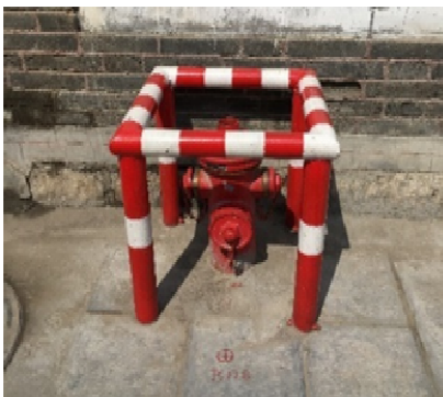
Fire hydrant in the upgraded street
