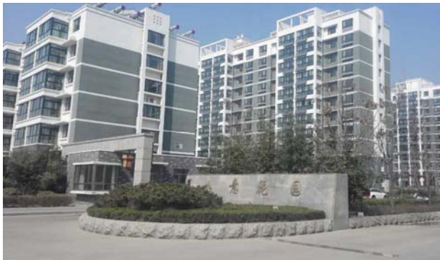
Resettlement housing for affected people from Gupan Pond area
