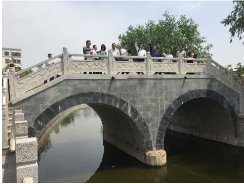
Bridge across Yinli River
