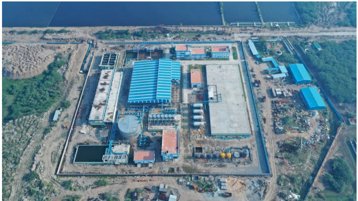
PHOTO 1. Tertiary Treatment Plant at Kodungaiyur
