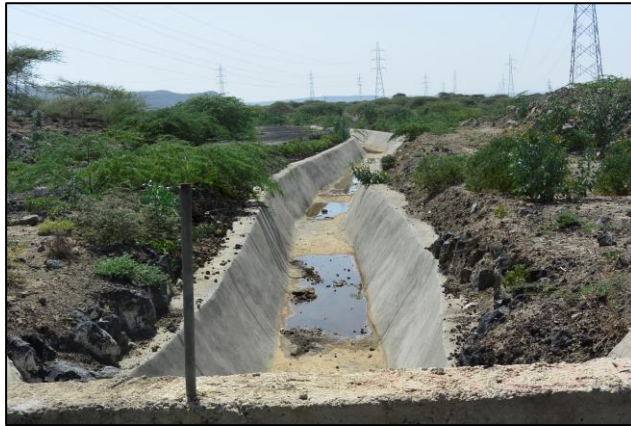
Figure 29: The irrigation canal of the Fentale Irrigation-Based Integrated Development Project. The left picture shows the sealed upstream section close to the existing high-voltage transmission lines while the right picture shows the excavated canal adjacent to the original project site.
