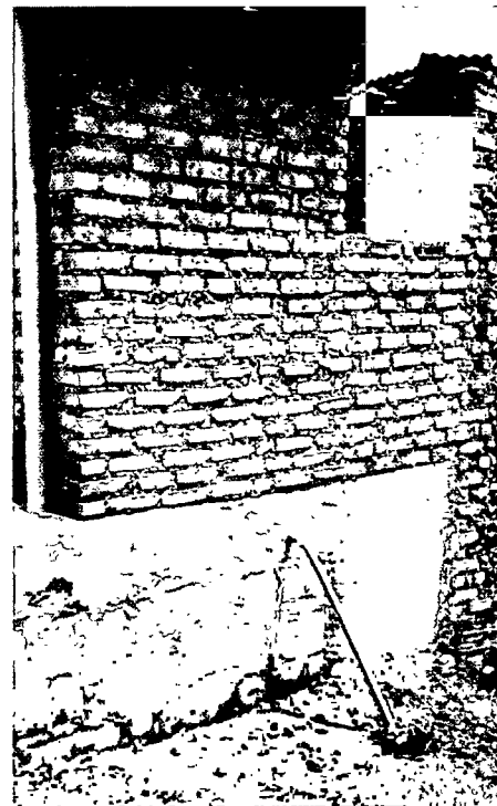
An option for hard rocky (fissured) terrain where excavating cost can be prohibitive and pit latrines lead to pollution of springs. (Kisoro, Uganda)
