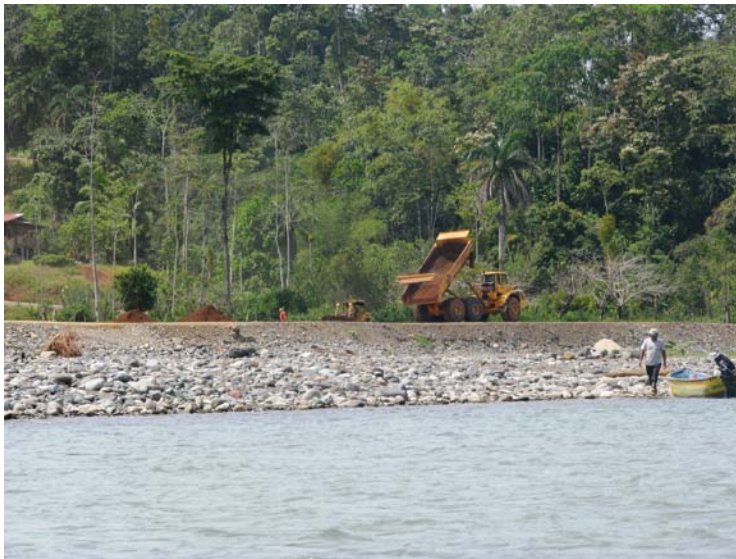
Picture 3 Road Construction along the Teribe River
