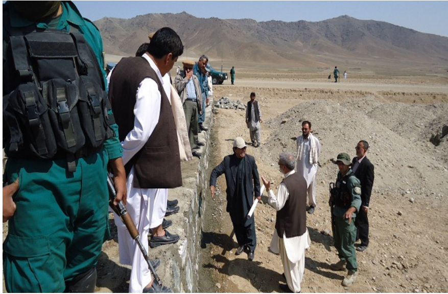
Picture7: Construction of Mosque at Resettlement Site
