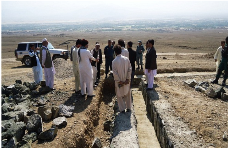
Picture 6: Deputy Minister inspecting quality of construction work at resettlement site
