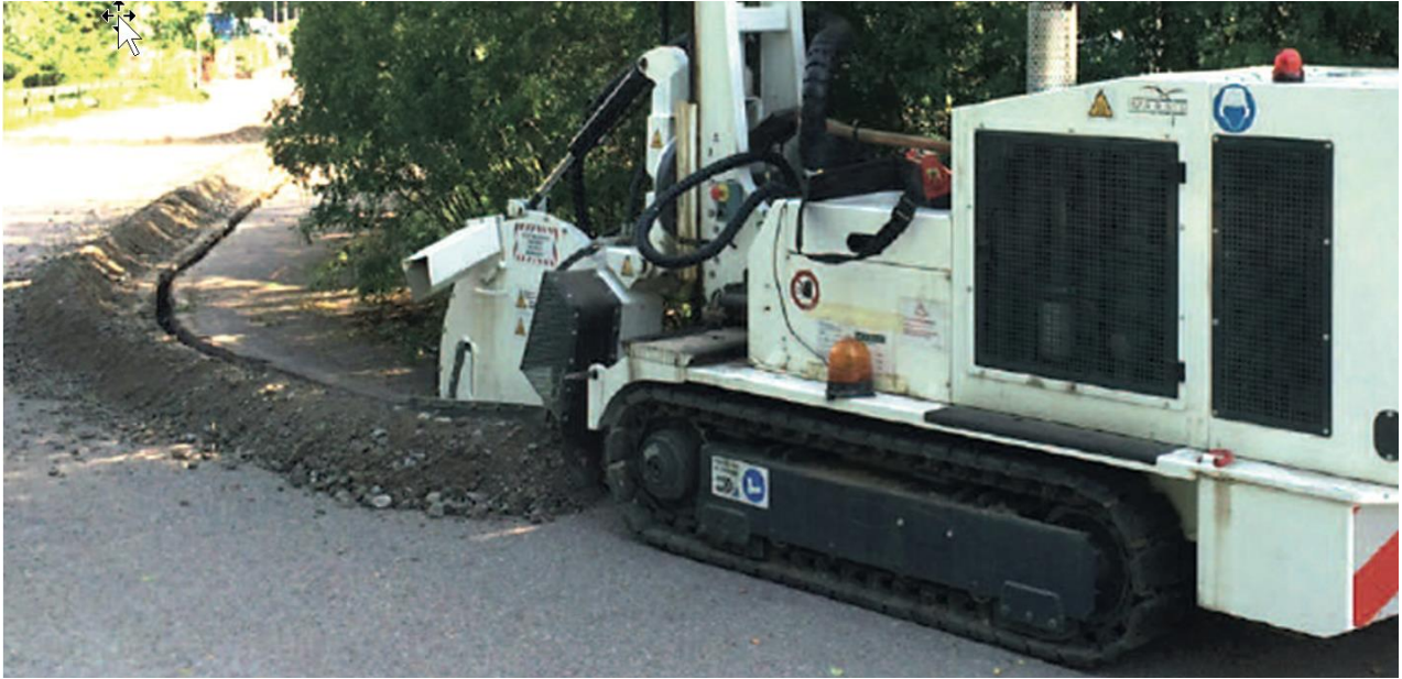
Figure 24- Marais Sidecut SC3C is an example of a microtrenching technology. It can achieve 500m per day in a wide range of terrain. 200km of fiber optics has been deployed in New Zealand by Marais to date. This equipment would be suitable for both Majuro and Ebeye environments.
