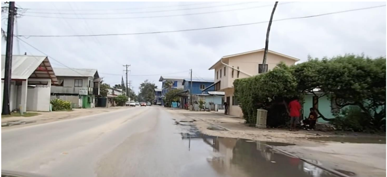
Figure 22 - Much of Majuro is an urban environment with hard surfaces that will require digging and reinstatement to both install the communal network and the individual connection to each home or business.
