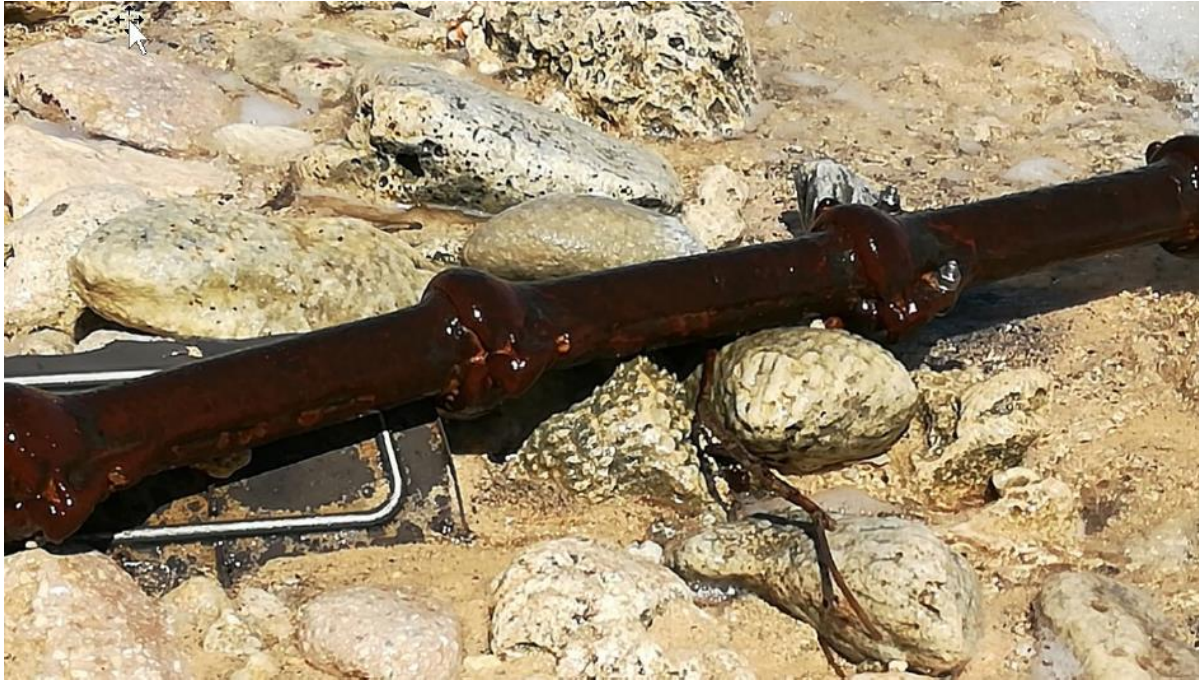
Figure 21 - Articulated Pipes at the landing, showing high erosion and cable in suspension
