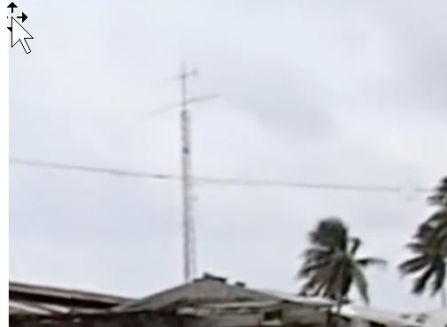
Figure 18 - HF Radio antenna on Majuro
