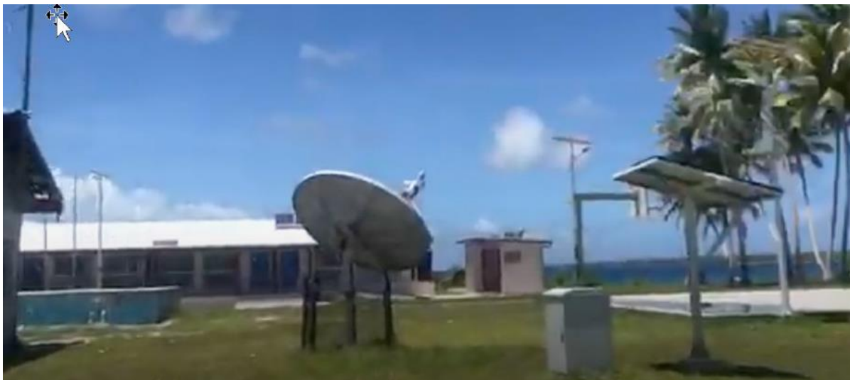
Figure 19 - Example of existing DAMA Satellite infrastructure in Ailinglaplap.
