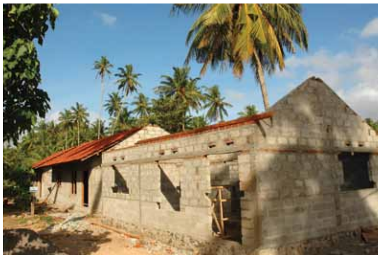
Bank support for post-Tsunami reconstruction in Aceh, Indonesia (2007)
