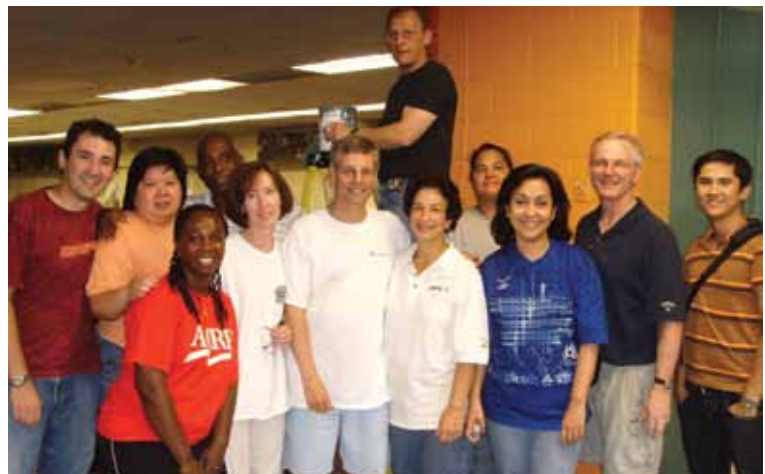
Bank staff volunteers installing student resource center in low-income high school in Washington, DC (2008)
