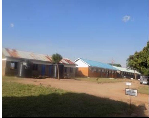
Photo 5: Apyeta Primary school in Lamwo District
