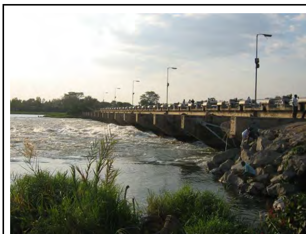
Figure 2. Downstream view of Kamuzu Barrage on the Shire River, Liwonde.
