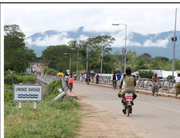
Figure 3. Kamuzu (Liwonde) Barrage road deck.
