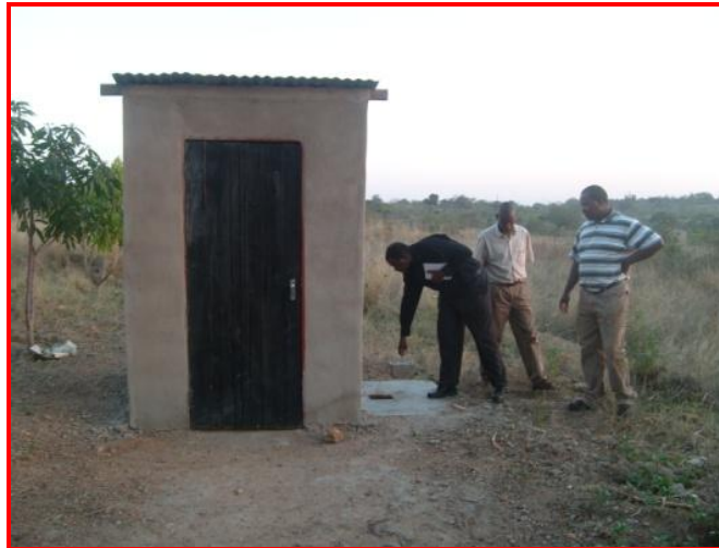
Figure 4-15 Concrete lined pit for Home based Health Care Waste
