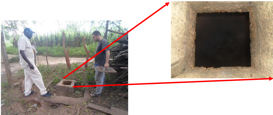
Figure 4-11 Concrete lined pit for sharps disposal at a Clinic
