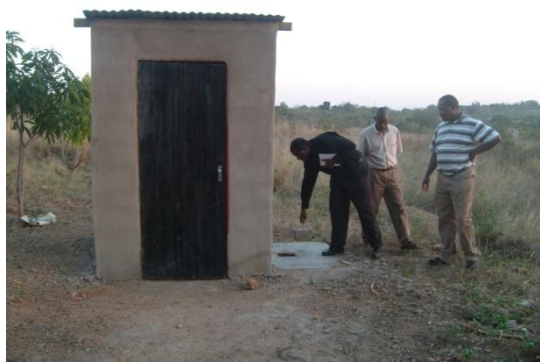
Pit with Pit Latrine for home based care
