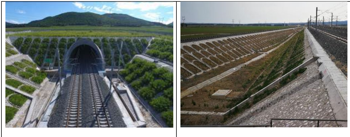
Figure 8. Good Environmental Protection Practices: Slope Protection
