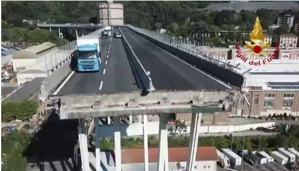
PHOTO 3.1 AERIAL PHOTO BY UAV, BRIDGE COLLAPSE - GENOA, ITALY
