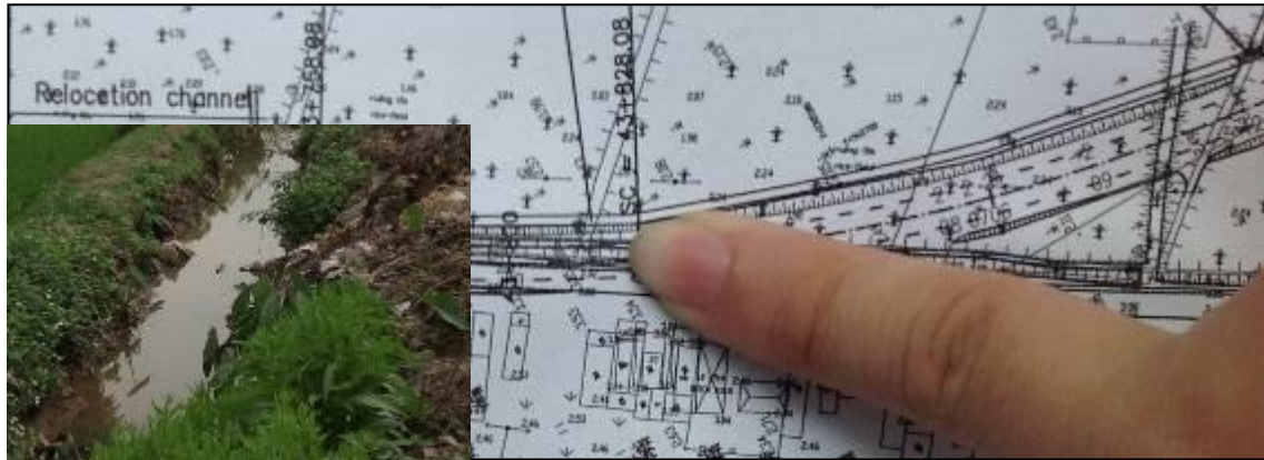
Irrigation Canal Km43+650
