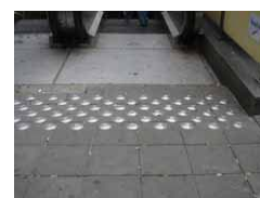
Rubber warning blocks at directional intersection
