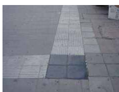
Concrete directional blocks
