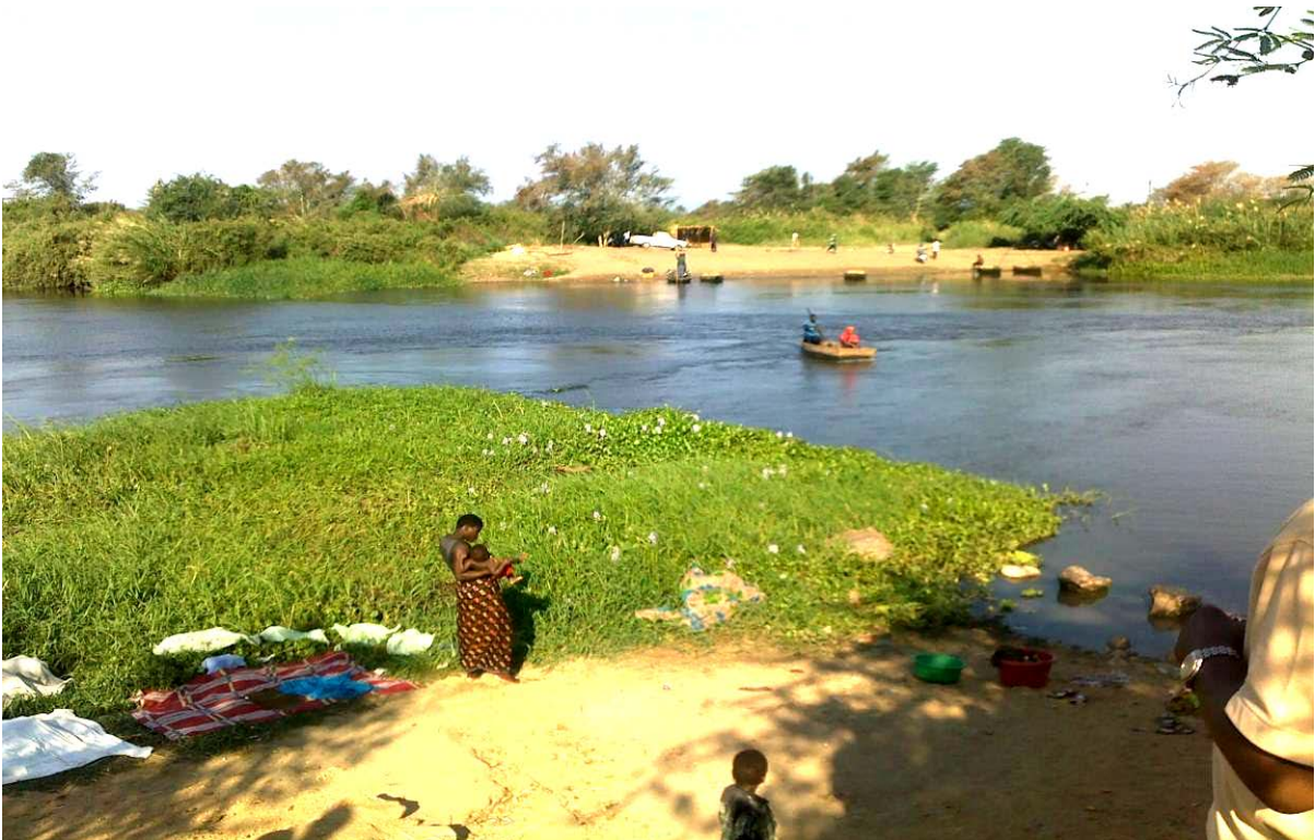
Fig. 2.19: A breached road connecting Bangula and Makhanga on the Shire River, Feb. 2012
