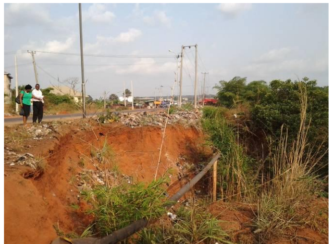
Plate 14: Gully Erosion Site close to Nnsukka High way
