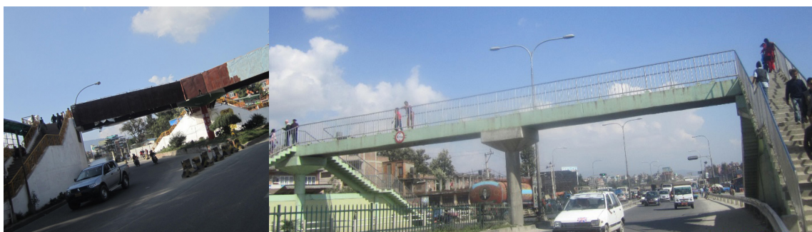
Enclosed bridges are a security hazard. The newer more open design footbridge below (in Bhaktapur) is much safer
